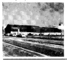
enclosed with vinyl-coated nylon tarp and polyethylene. Khapra adults, larvae, and eggs were spotted in test cages throughout the building. About one mile of Saran tubing strung about the interior permitted continuous monitoring of fumigant concentration at strategic points during the test.
